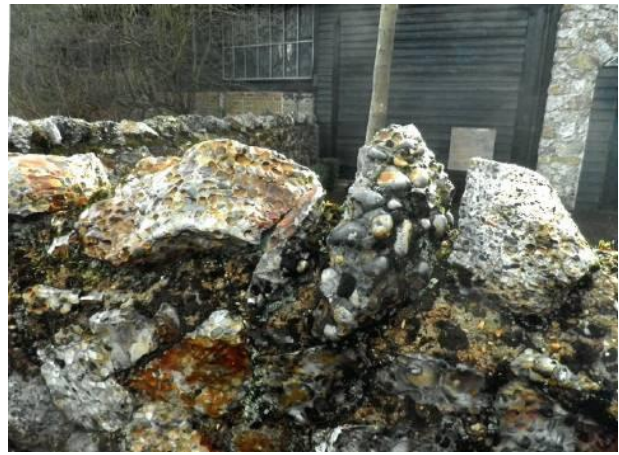
Farm wall built entirely of local cobble-size puddingstone near Battlers Green.
